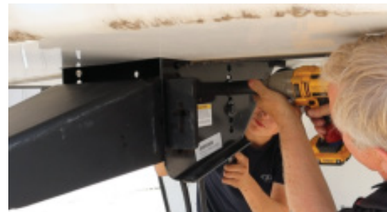
Figure 2: Install safety chain bracket onto pin box frame
