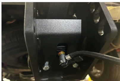
Figure 16: Filling up air spring bag using an air compressor on the valve stem
