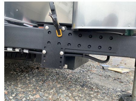
Figure 2: Clamp-on hardware added loosely
