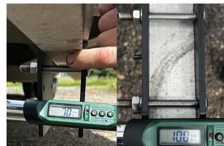
Figure 8: Left Image: Bottom bolts have a gap so torqued to 7 ft-lbs Right Image: Top bolts torqued to 10 ft-lbs
