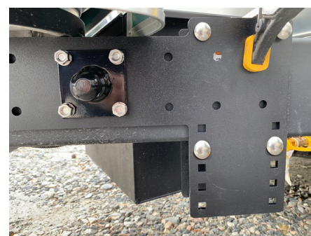
Figure 7: All hardware added and tightened
