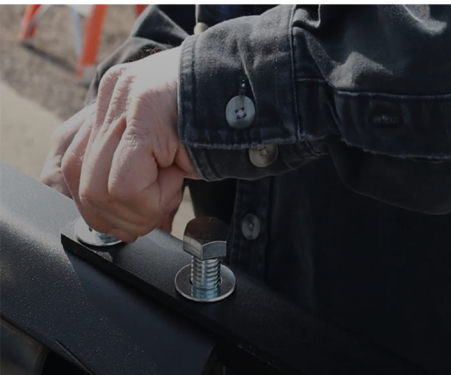
Figure 4: Use (4) 5/8" x 1 1/2" hex bolts & (4) 5/8" washers, on top studs. Finger tighten
