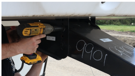
Figure 1: Unbolt your existing 5th wheel pin box
